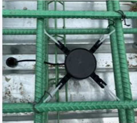
Sensor installed at Deck
